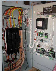
Switchgear, Relays, & Controls
